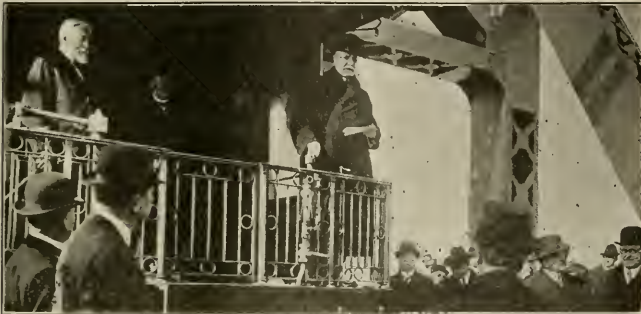
PRESIDENT SAMUEL REA DEDICATING THE HELL GATE BRIDGE AND THE NEW YORK CONNECTING RAILROAD. GUSTAV LINDENTHAL, DESIGNER OF THE BRIDGE, ON THE LEFT.
